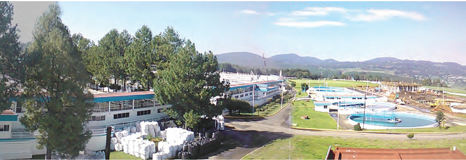
The drinking water treatment plant in Cutzamala.
